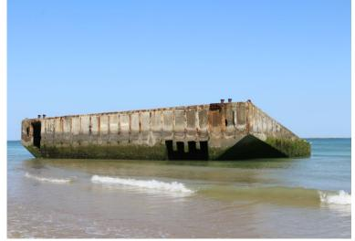
These were huge sections of floating concrete roads dragged across from Britain and fastened together at Arromanches forming a temporary harbour for ships to unload their cargo in support of the soldiers who had recently landed on the beaches. Over 19 million tonnes of supplies were offloaded at the Mulberry Harbour of Arromanches.
